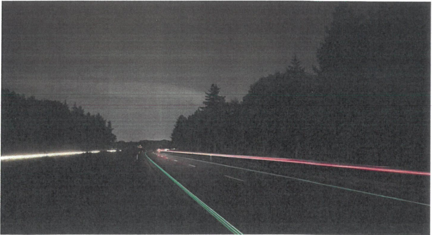
A road in the Netherlands has had glow-in-the-dark markings painted onto it for increased visibility and safety
