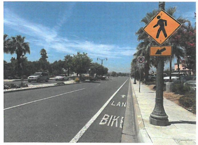
Class II bike lane on Base Line.
