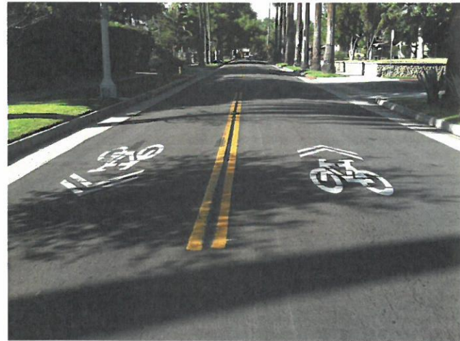
Class III facilities provide bike routes on low-speed streets.
