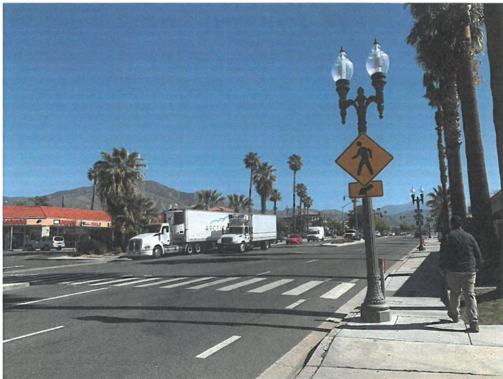
A high-visibility crosswalk enhances the visibility of pedestrians at this crossing on Base Line at Reedy Avenue. In-street lights, activated with a push button, further alert vehicles of a pedestrian's presence at the crosswalk.
