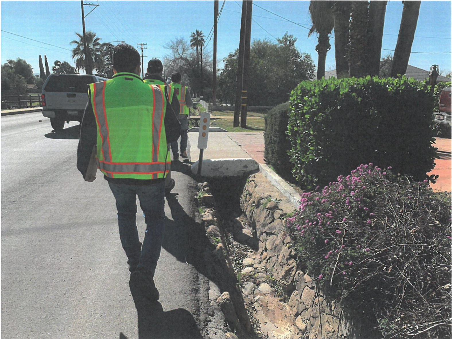
Much of the western side of Palm Avenue between Main and Messina Streets lack sidewalks.
