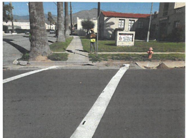
Crossings without curb ramps (such as this one on Main Street and Palm Ave) present difficult conditions for children, older adults, and people using wheelchairs, strollers, or other mobility devices.
