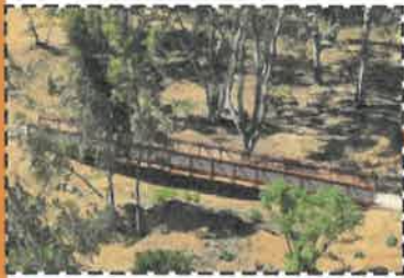
Install New Prefabricated Pedestrian Bridge for Wash Crossing (Optional/ Recommended)
