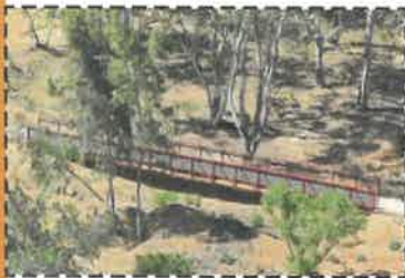
Install New Prefabricated Pedestrian Bridge for Wash Crossing (Optional/Recommended)
