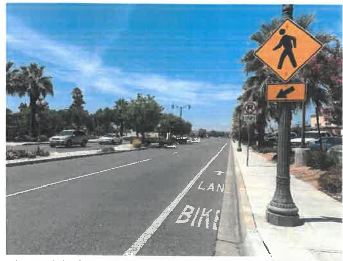
Class II bike lane on Base Line Street.
