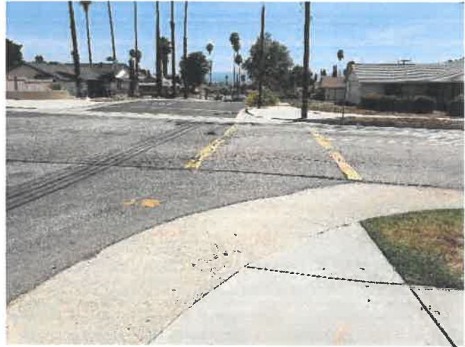
Crosswalks near schools, such as these by Highland Pacific Elementary, are marked yellow.
