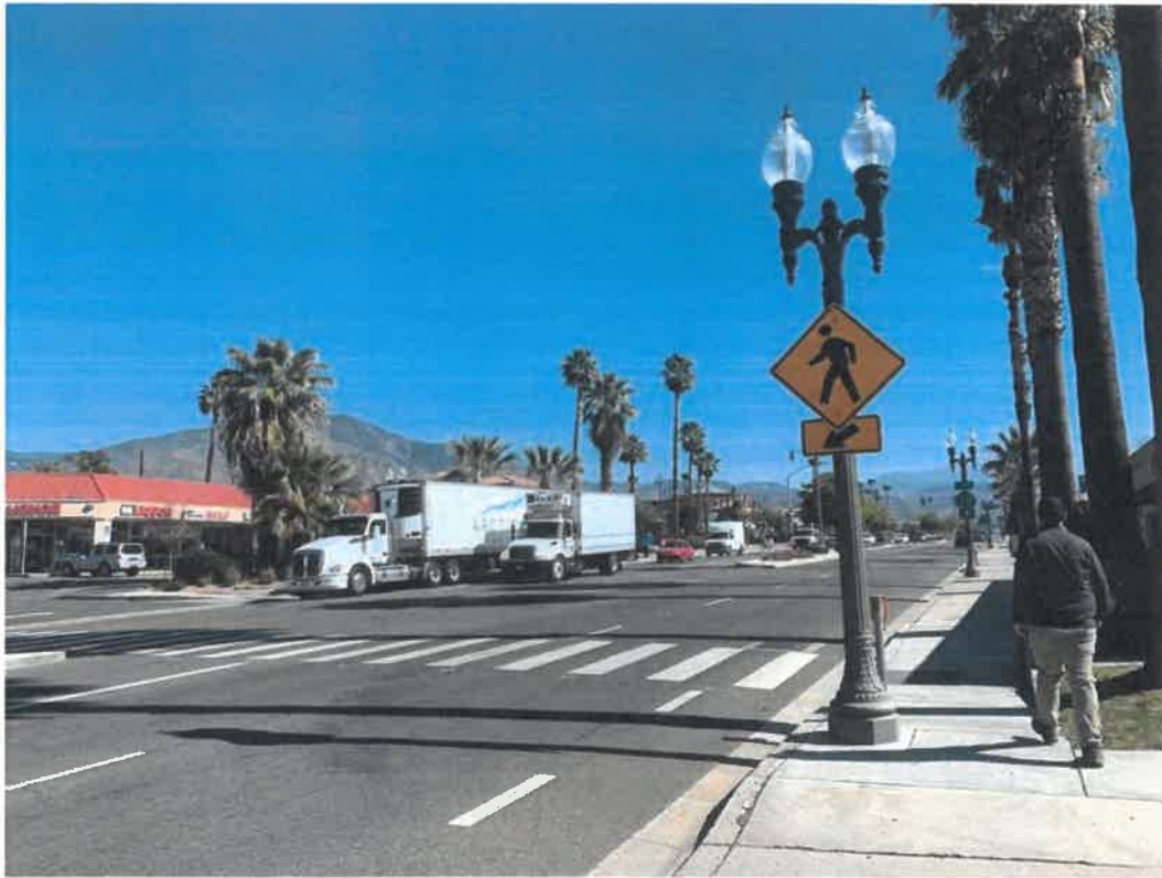
A high-visibility crosswalk enhances the visibility of pedestrians at this crossing on Base Line Street at Reedy Avenue. In-street lights, activated with a push button, further alert vehicles of a pedestrian's presence at the crosswalk.
