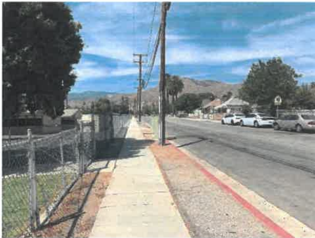
Sidewalk on Orange Street near Highland Pacific Elementary School.
