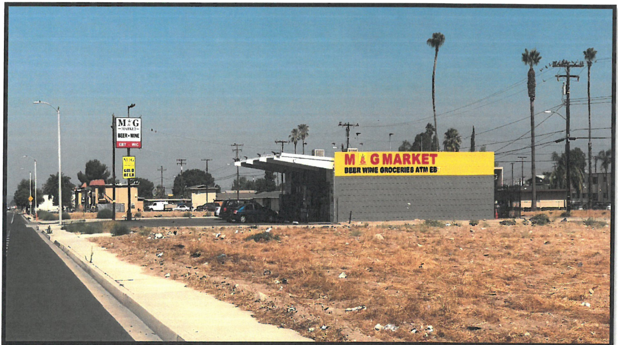
Right Side of the Store (East Side)
