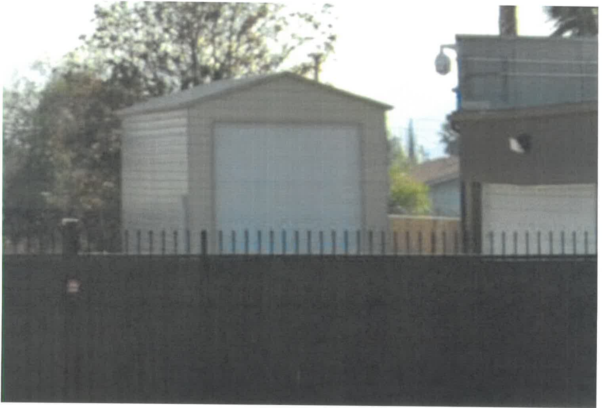
Existing Unpermitted Storage Building at SW Corner to be Demolished
