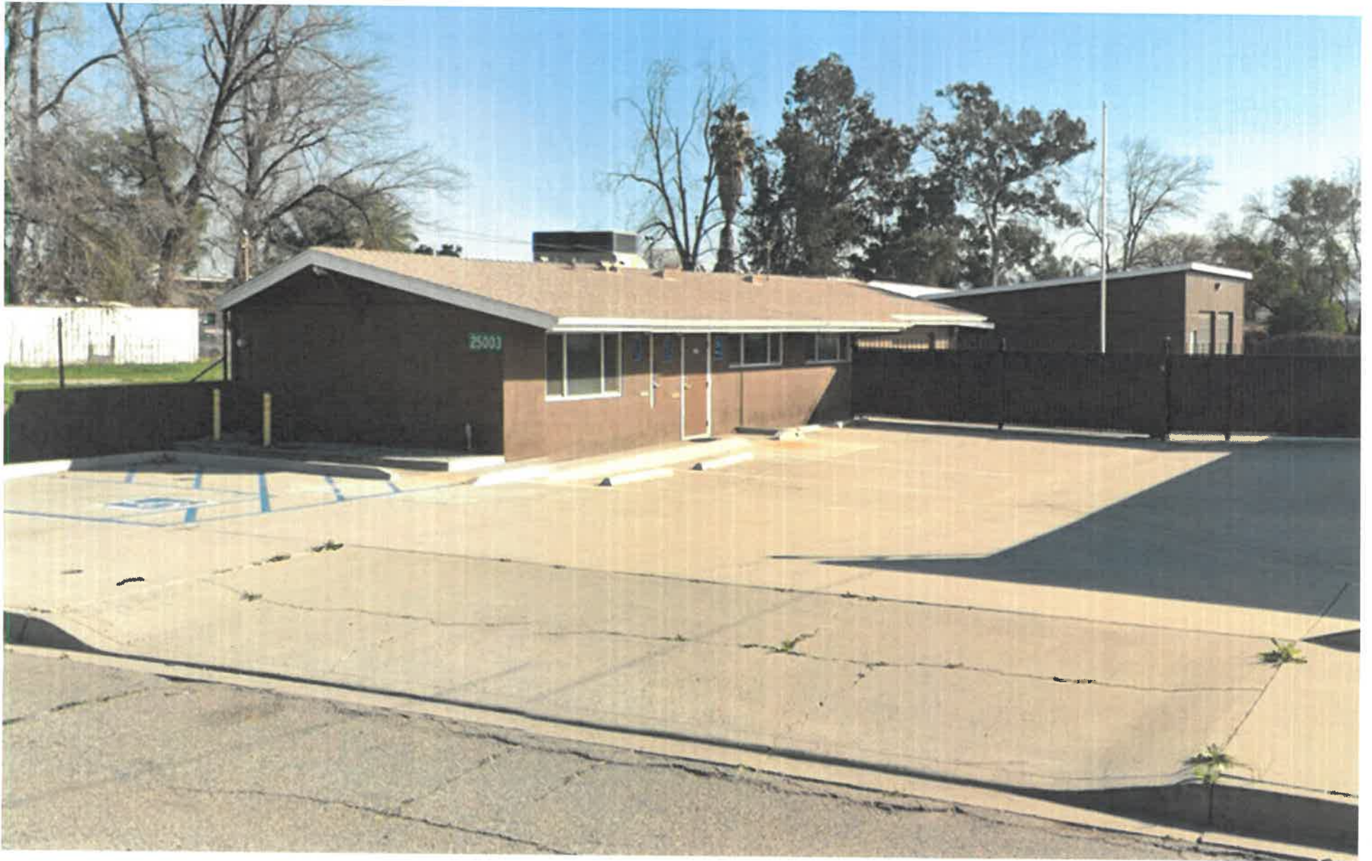
Existing Office Building at NE Corner to Remain
