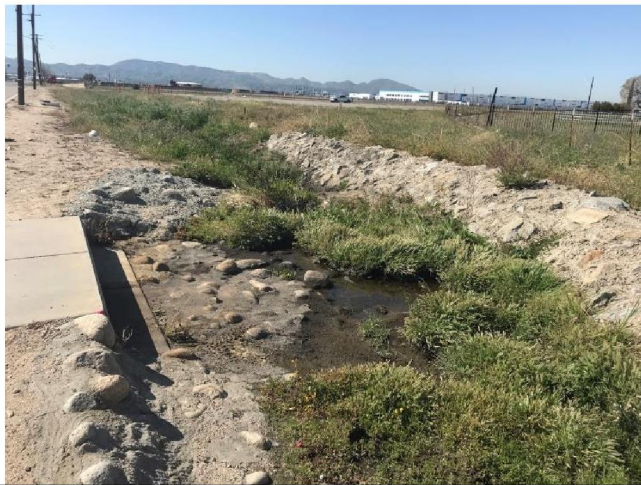
Photo Point 1: Facing south. Displaying northern inlet.
