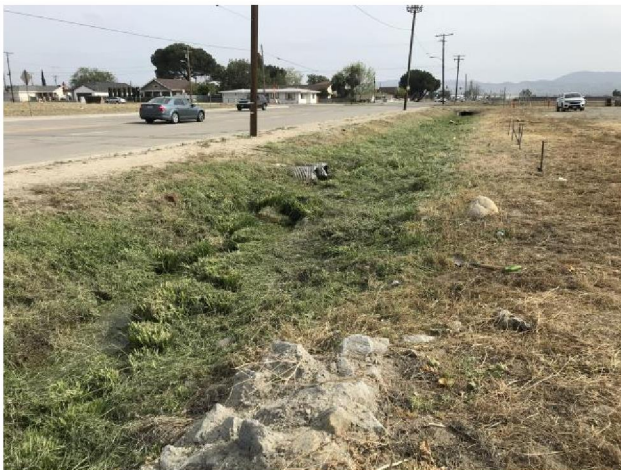
Photo Point 3: Facing Southeast. Upland drainage facing downstream with two culvert inlets in background.
