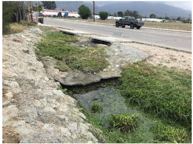
Photo Point 2: Facing north. Northern most portion of the channel with concrete rip rap on banks.
