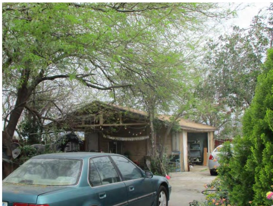
Figure 2. Parcel 1 garage, south elevation, view looking northwest (IMG_6057)
