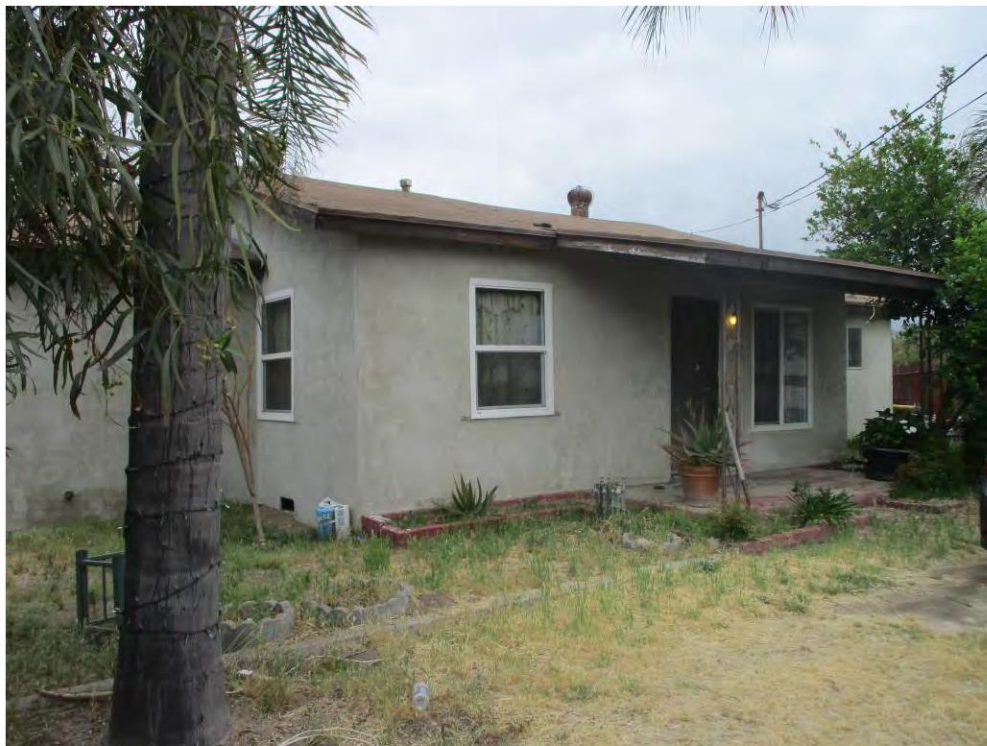
Figure 1. Parcel 1 single-family residence, East (primary) elevation, view looking northwest (IMG_6053)
