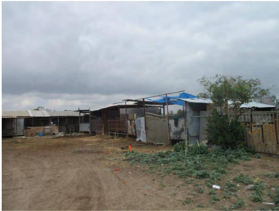
Figure 8. Parcel 1 horse barns, view looking northwest (IMG_6073)
