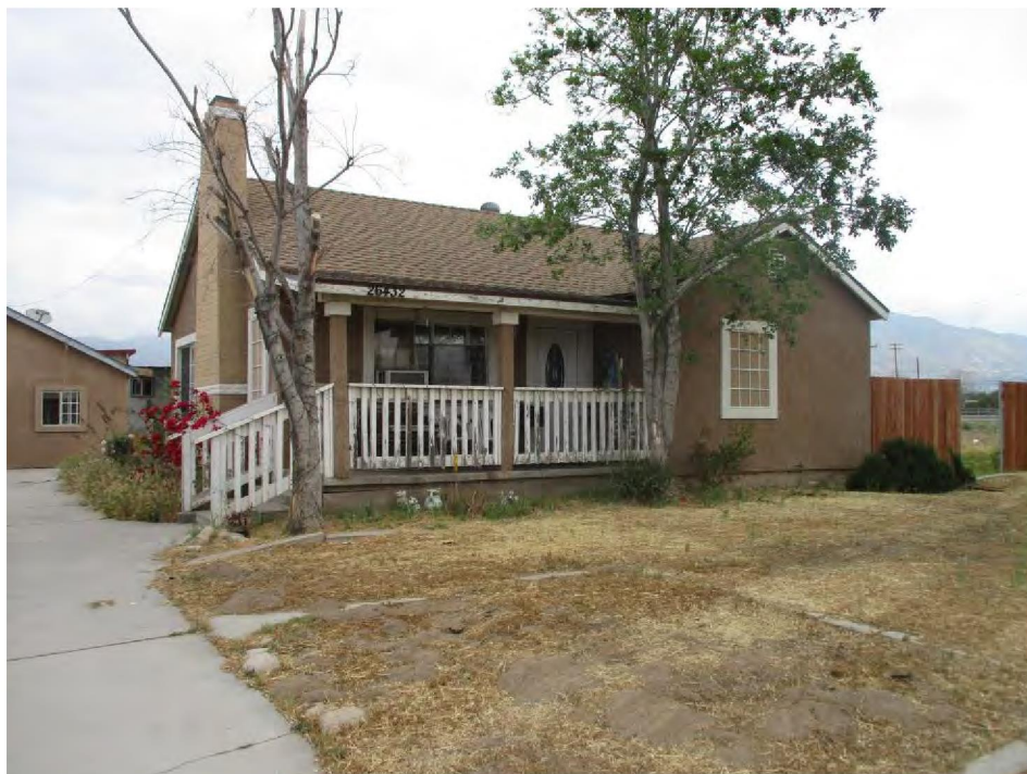
Figure 9. Parcel 2 single-family residence, south (primary) elevation, view looking northeast (IMG_6190)
