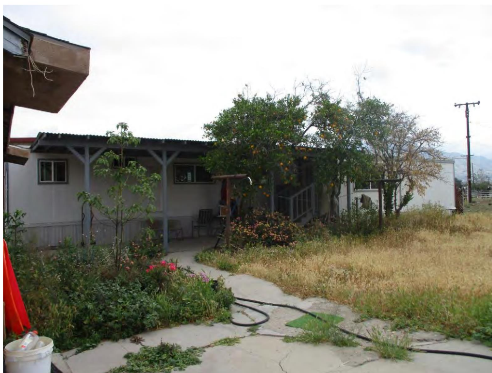
Figure 10. Parcel 2 mobile home, south elevation, view looking northeast (IMG_6194)
