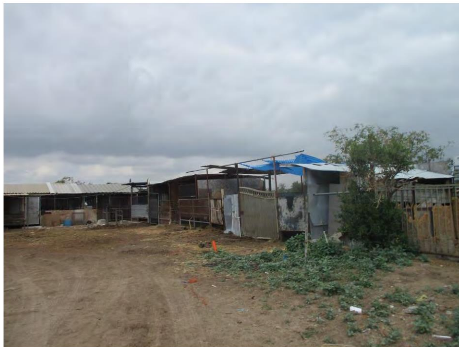
Figure 3. Parcel 1 horse barns, view looking northwest (IMG_6073)
