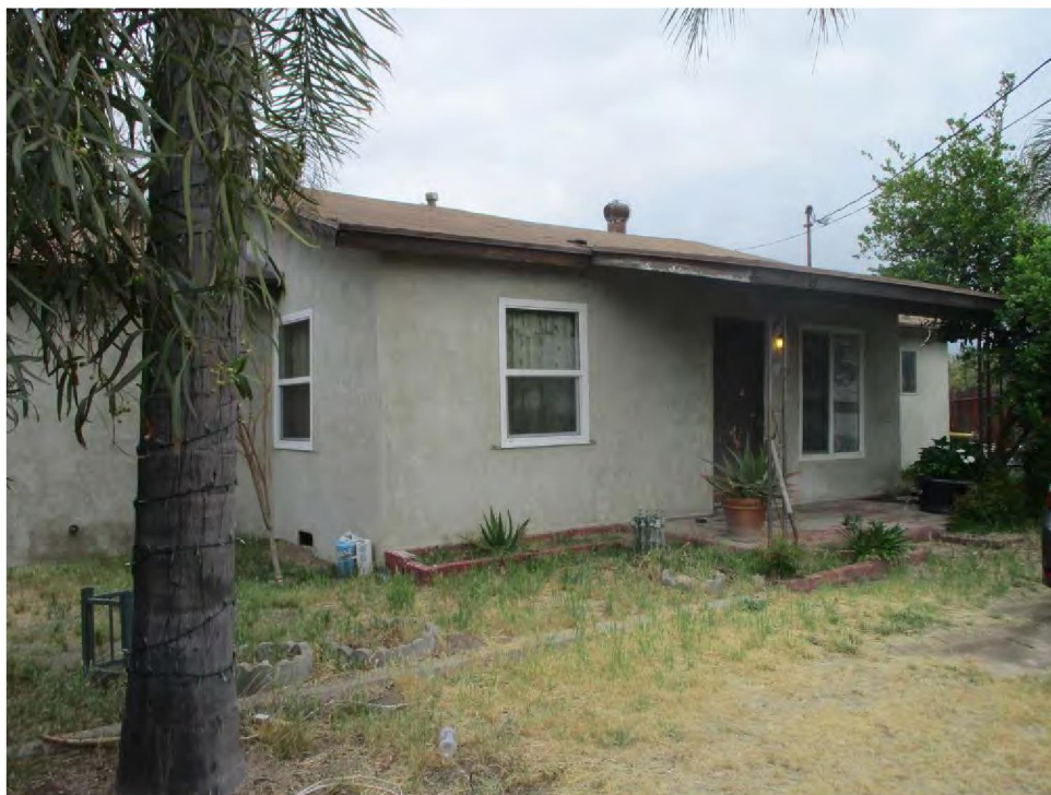
Figure 6. Parcel 1 single-family residence, East (primary) elevation, view looking northwest (IMG_6053)
