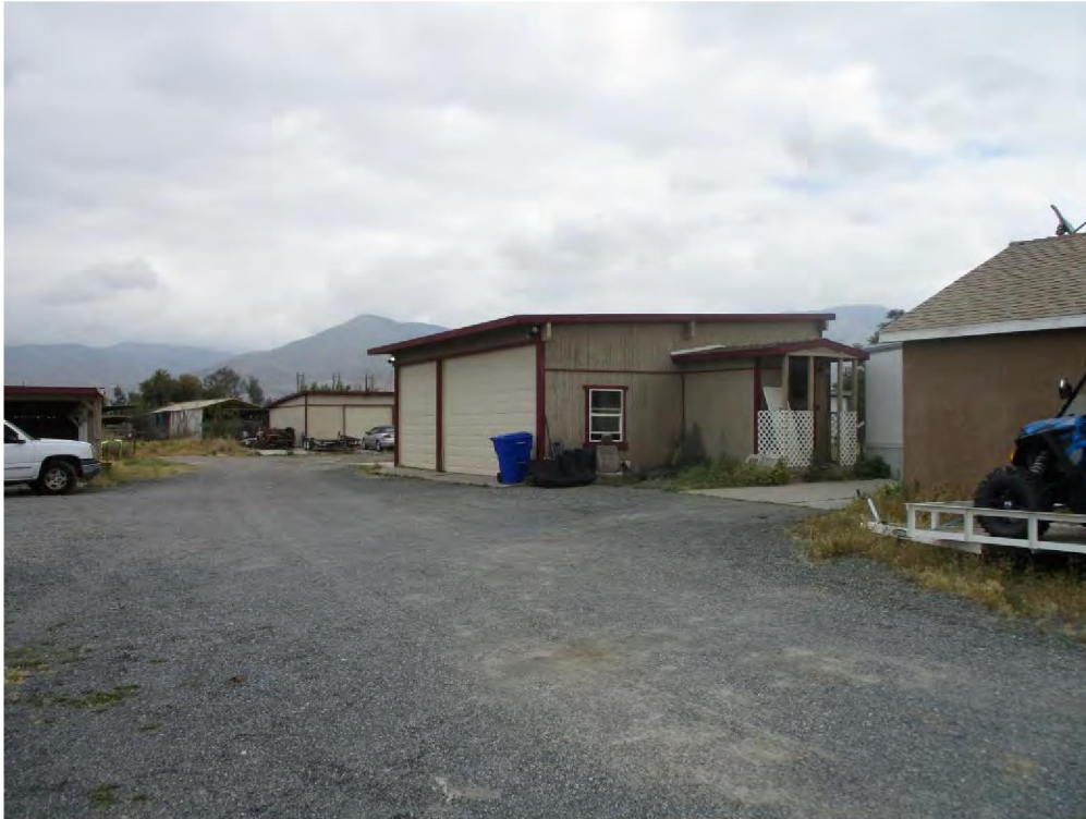
Figure 11. Parcel 2 garage south elevation, view looking northeast (IMG_6204)
