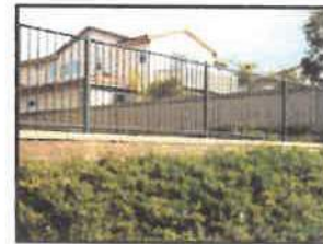
② Perimeter View Fence
