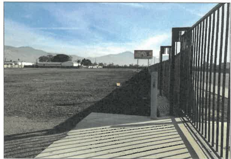
Photo A: From the southwest corner of the project site, facing east. Representative of the crumbling asphalt covering most of the project site.
