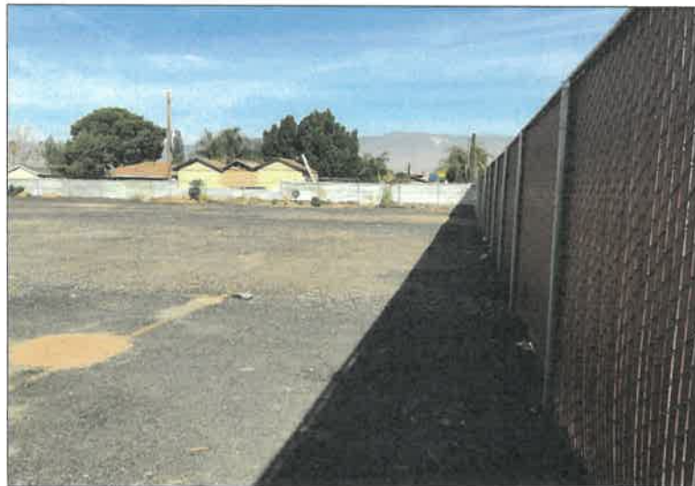
Photo E. From the southeastern corner of the project site, facing north.
