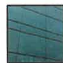
D. STOREFRONT MEDIUM PERFORMANCE BLUE REFLECTED GLAZING BLACK ANODIZED MULLION
