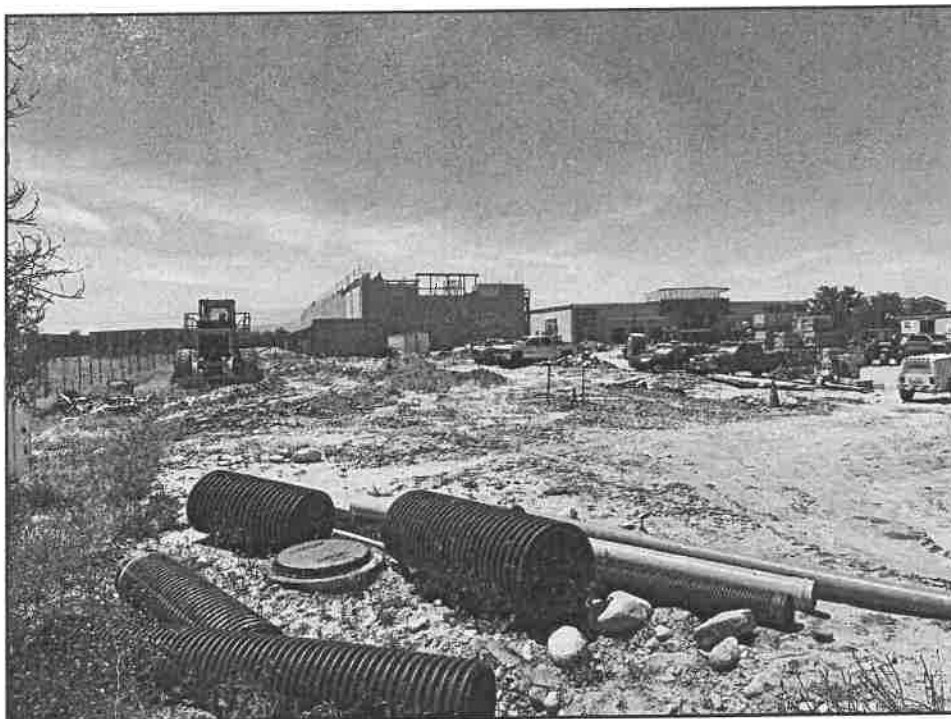
Photo 4: Northeast corner of Project site, looking south.
