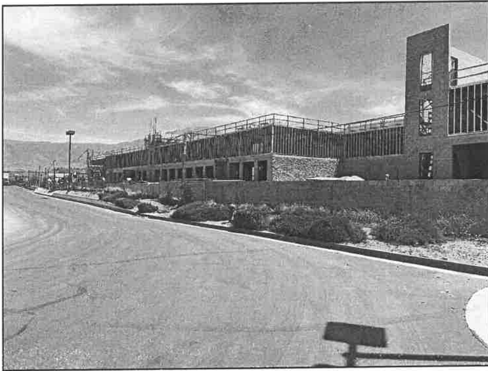
Photo 1: Southwest corner of Project site, looking northeast.
