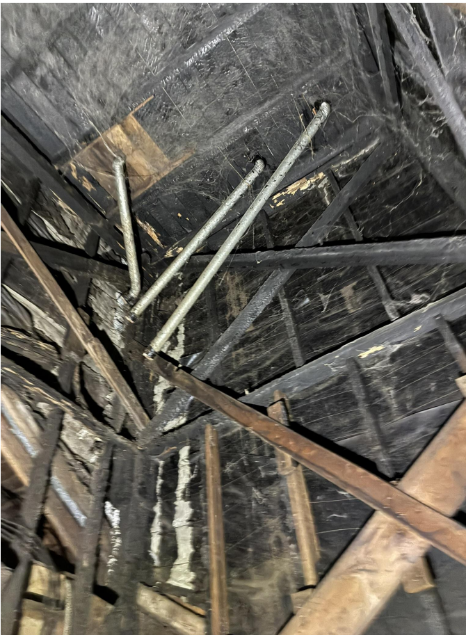
FIGURE 11. FIRE DAMAGE AT SOUTH BELL TOWER WALL
