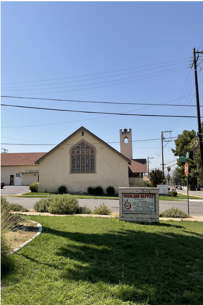
FIGURE 5. VIEW OF THE NORTH FACE OF TOWER
