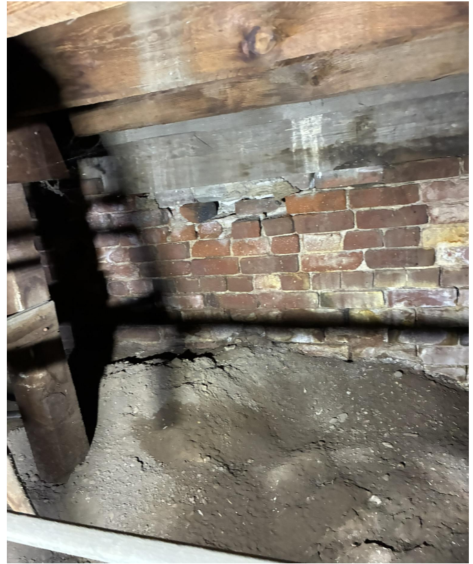
FIGURE 3. EXISTING FOUNDATION AT WEST WALL
