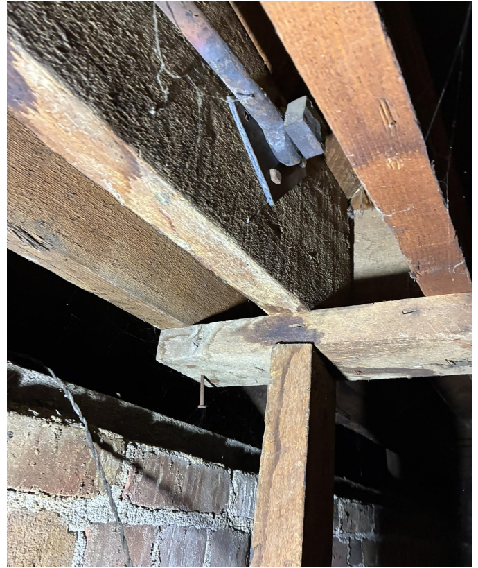
FIGURE 8. BEAM BRACING ROD END CONNECTION
