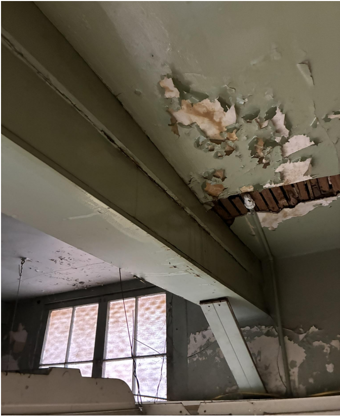
FIGURE 7. WEST END OF TOWER SUPPORT BEAM
