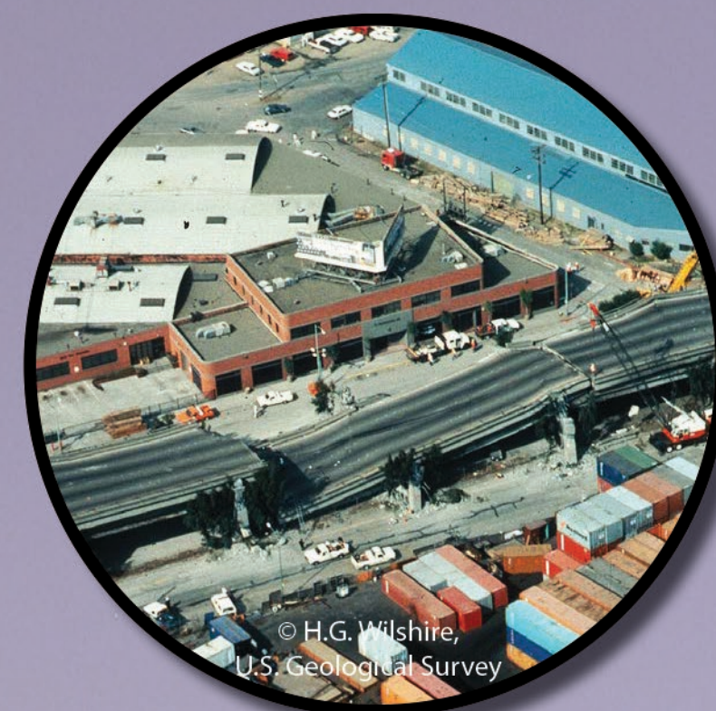
1989 LOMA PRIETA EARTHQUAKE
