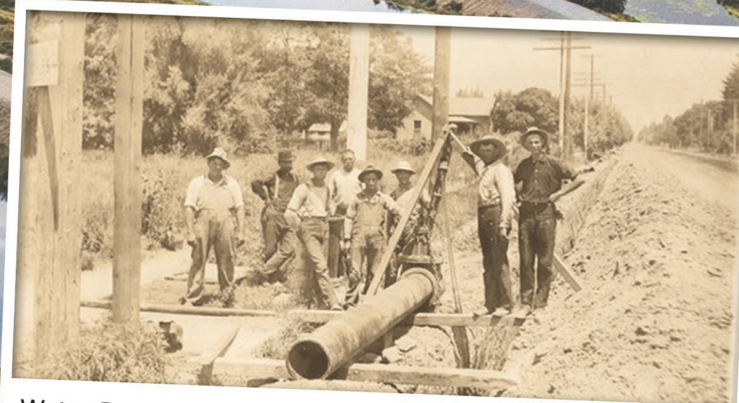
Water Department Crew laying out a pipe on 6th Street in the 1930s.
