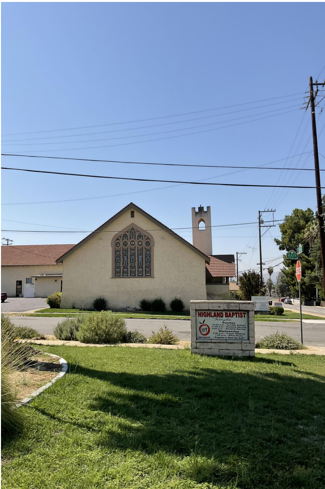
FIGURE 5. VIEW OF THE NORTH FACE OF TOWER
