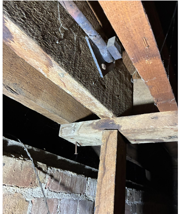
FIGURE 8. BEAM BRACING ROD END CONNECTION
