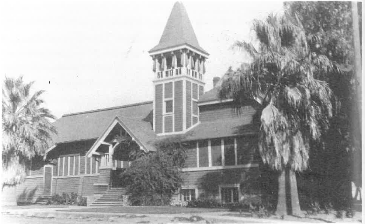
In 1947, an electrical wire caused a fire in the church, and two-thirds of the building burned. Take note of the steeple in this photo and the next.
