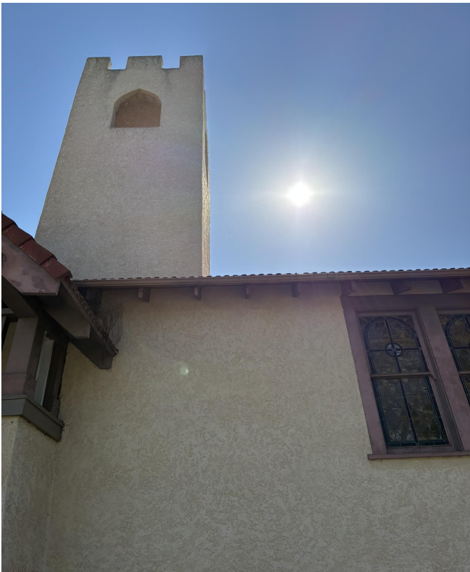
FIGURE 9. WEST TOWER VIEW
