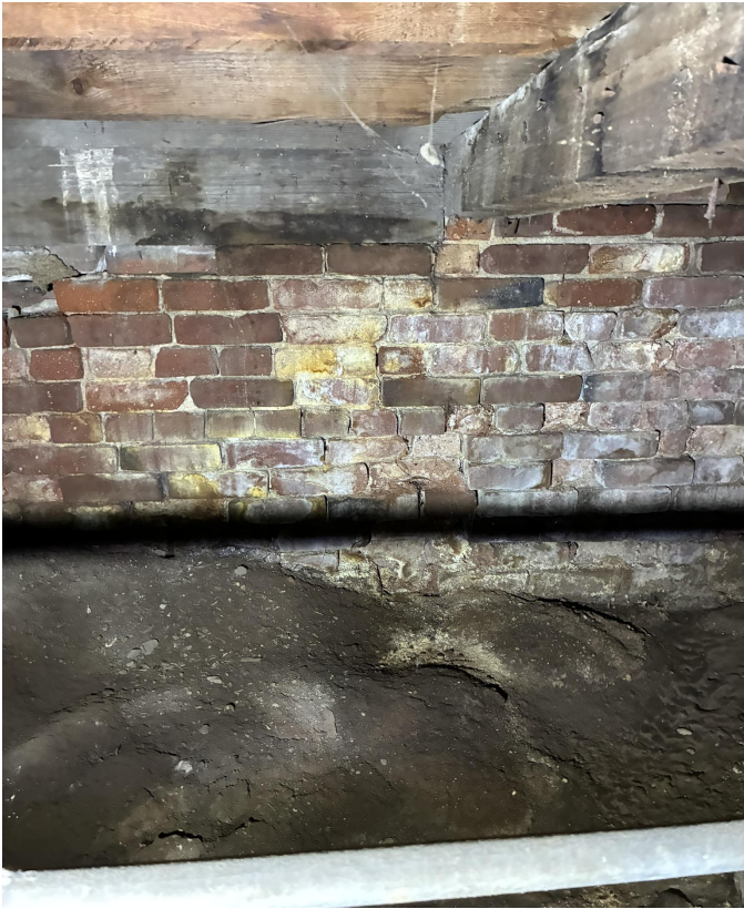
FIGURE 2. EXISTING FOUNDATION AT WEST WALL
