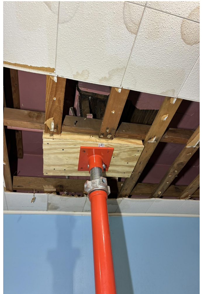
FIGURE 6. TOWER BEAM TEMPORARY SUPPORT INSTALLED IN BASEMENT
