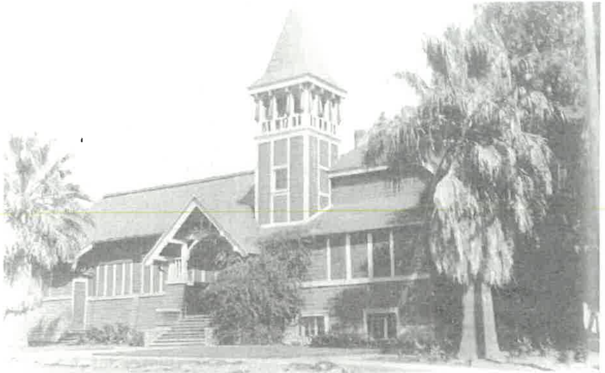
In 1947, an electrical wire caused a fire in the church, and two-thirds of the building burned. Take note of the steeple in this photo and the next.
