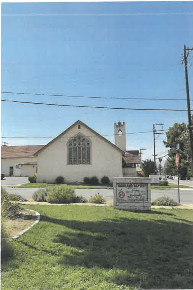
FIGURE 5. VIEW OF THE NORTH FACE OF TOWER
