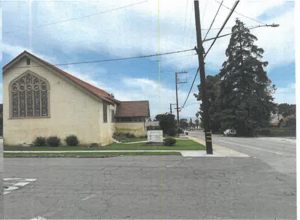
Church Without Bell Tower
