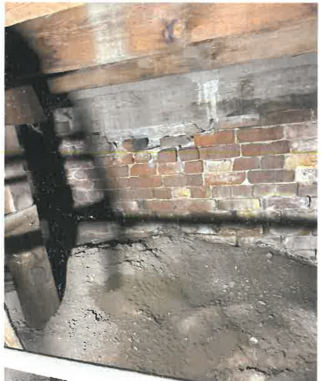
FIGURE 3. EXISTING FOUNDATION AT WEST WALL
