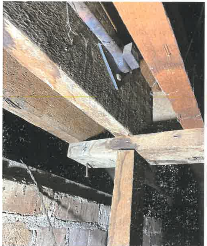
FIGURE 8. BEAM BRACING ROD END CONNECTION
