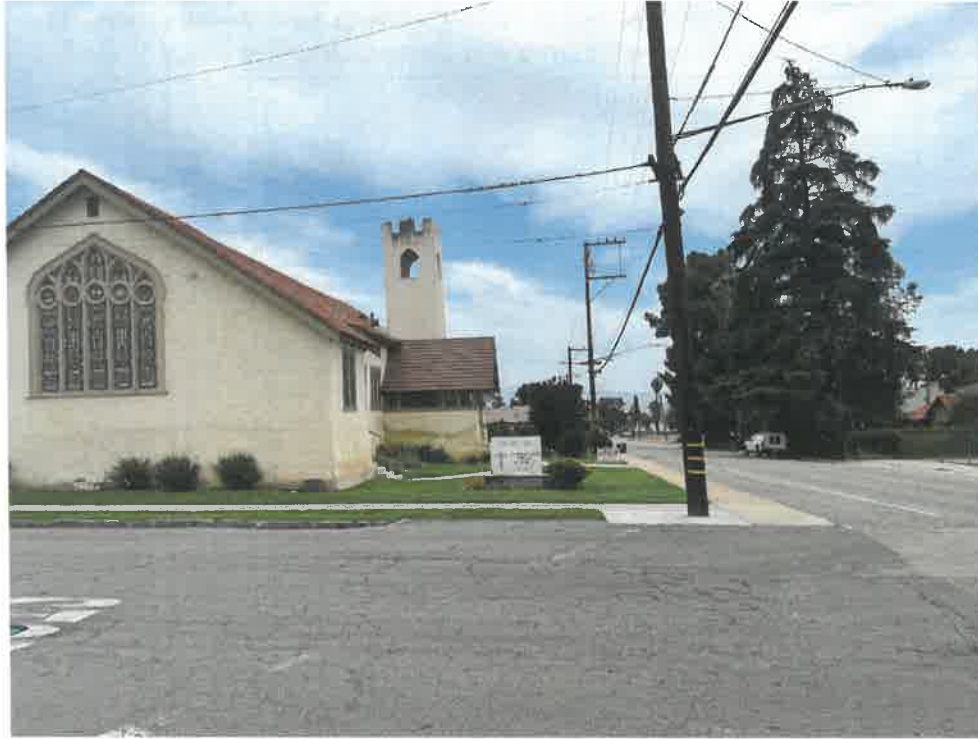
Church with Bell Tower
