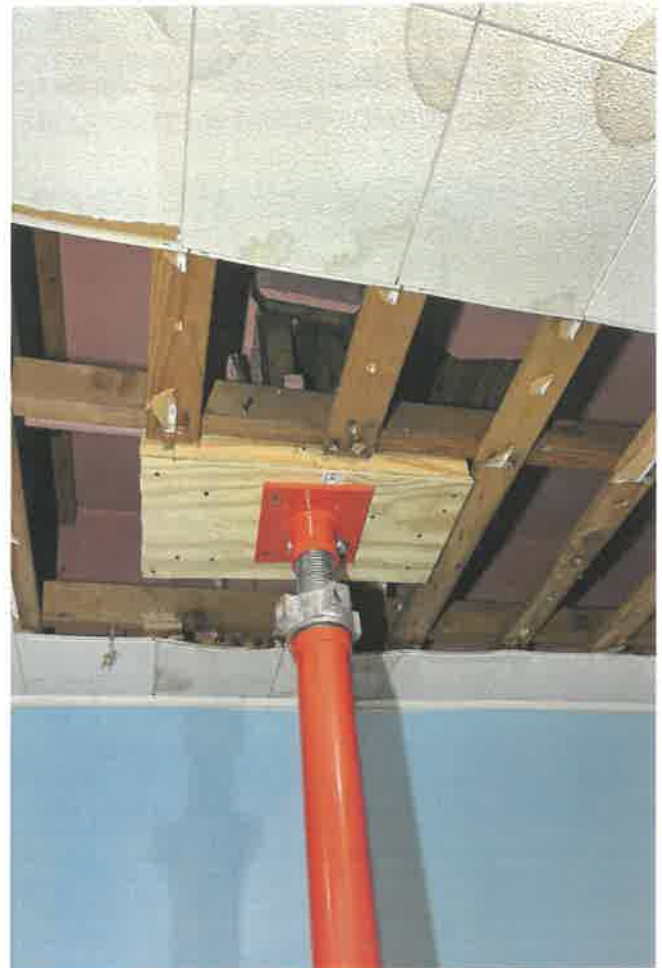
FIGURE 6. TOWER BEAM TEMPORARY SUPPORT INSTALLED IN BASEMENT
