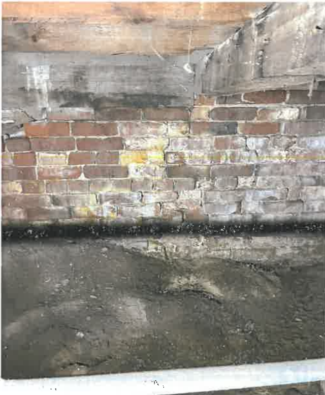
FIGURE 2. EXISTING FOUNDATION AT WEST WALL
