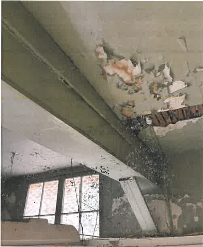
FIGURE 7. WEST END OF TOWER SUPPORT BEAM
