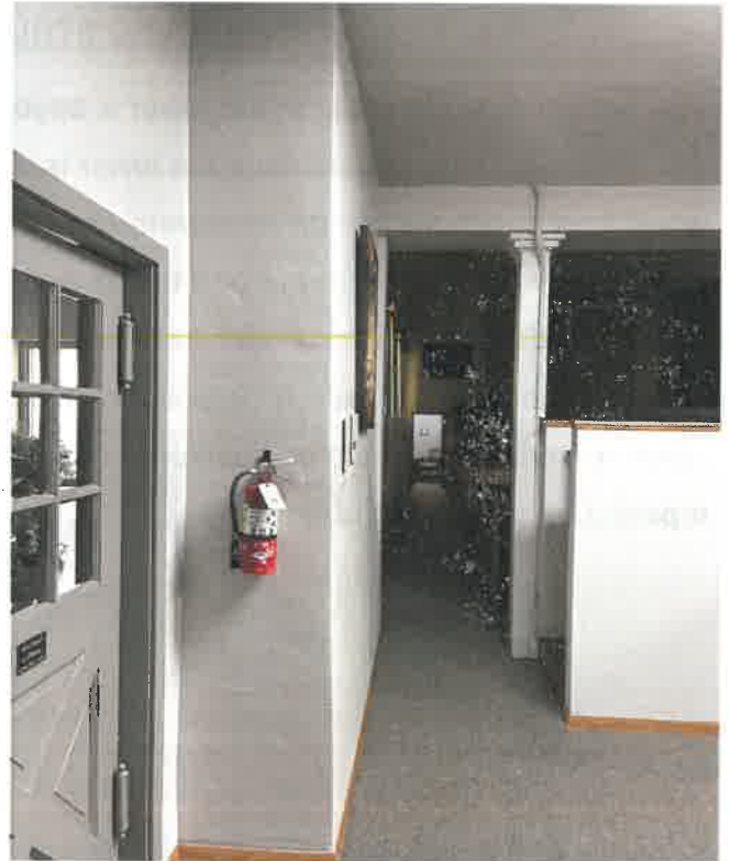
FIGURE 14. LOWER EAST SUPPORTING WALL
